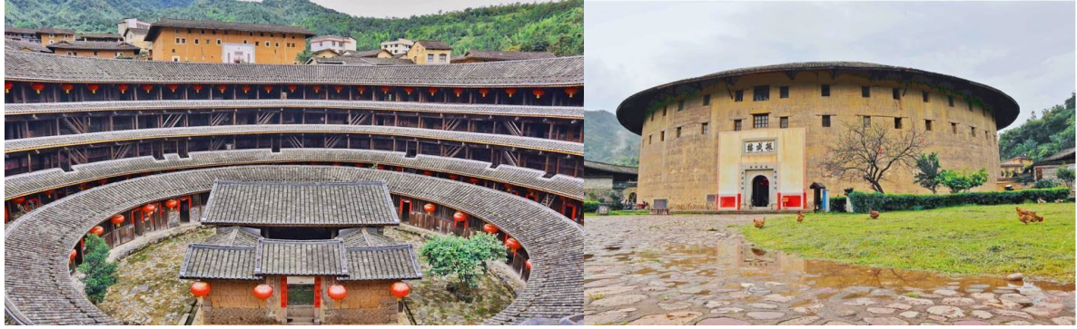
262 263 Fig 4. Example of tulou in Yongding © the first author 264
