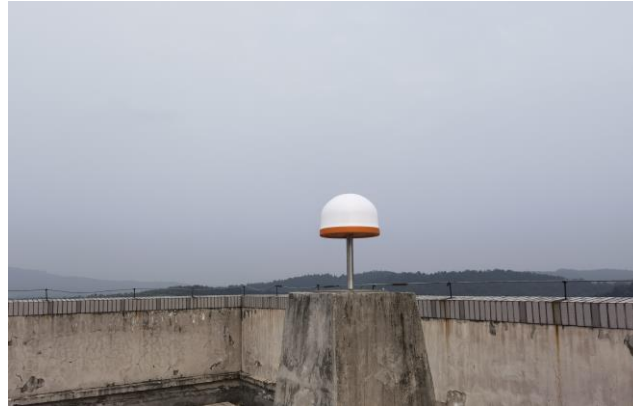
Fig. 14 Monitoring equipment No. 2 in an ideal environment
