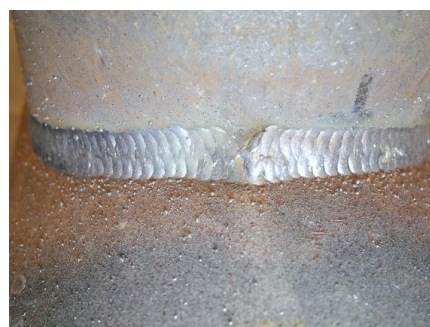
d) Welding quality at the brace-chord junction
