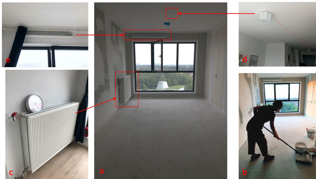
Figure 4. Interior of a typical apartment in the Dutch modular student housing. a) full view of the apartment; b) conducting furnishment in the apartment; c) radiator in the apartment; d) lightings in the apartment; e) ventilation grille in the apartment.
