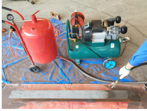
Fig. 3 Sandblasting of the steel surface
