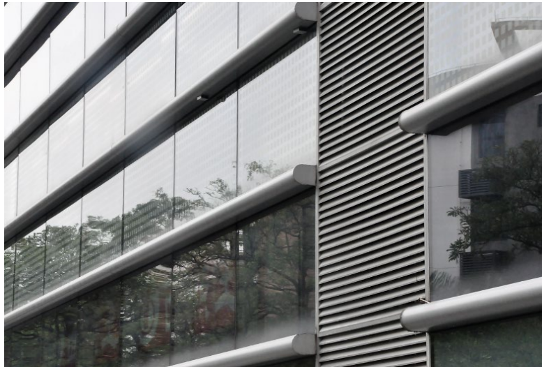
(b) Detail of facade decoration
