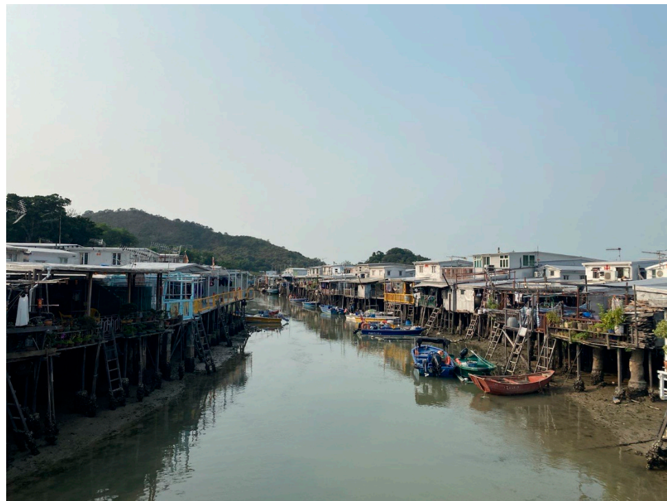
Figure 1. Stilt Houses in Tai O.
