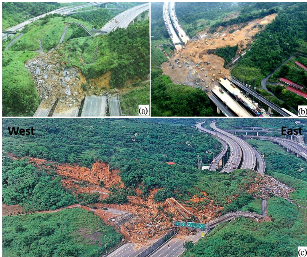
Figure 3. Aerial photos taken from site after landslide. (a) Photo from northeast direction; (b) Failure plane during the removal of debris; (c) Photo from south direction.
