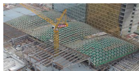
(a) Overall view
