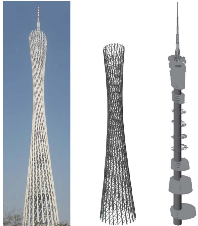
Fig. 1. Canton Tower: bird's-eye view, outer tube, and inner tube.
