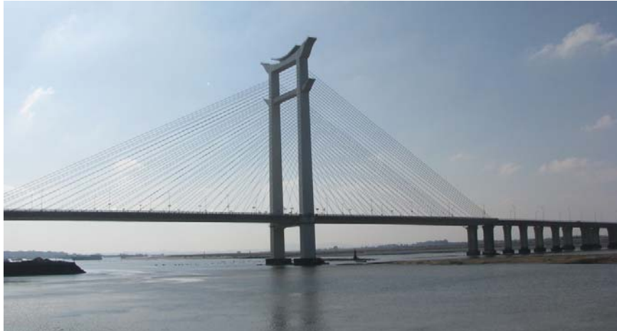
Fig. 2 View of the Jing Jiang Bridge
