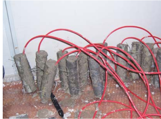
(b) Concrete coating
