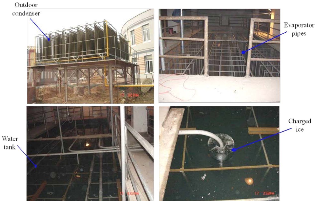
Fig.15 Implementation of the seasonal cold storage system
