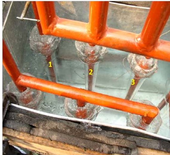
b. Charged ice in the storage tank
