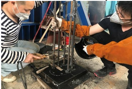
(a) Welding longitudinal rebars to the bottom steel plate
