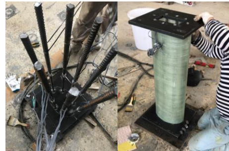
(b) Placing the FRP tube and the top steel plate
