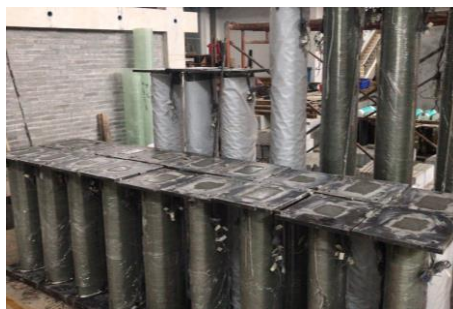
(e) Casting the concrete
