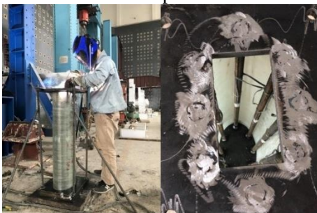
(c) Welding the longitudinal rebars to the top steel plate
