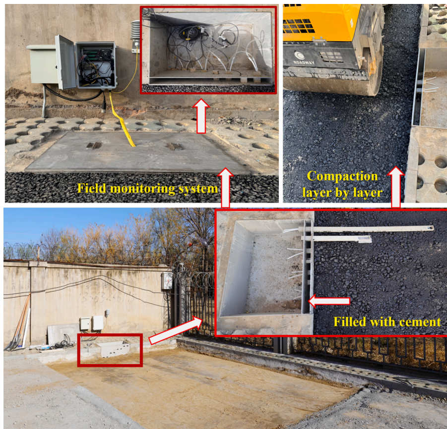
Fig. 9. The field construction process and the layout of the monitoring system.
