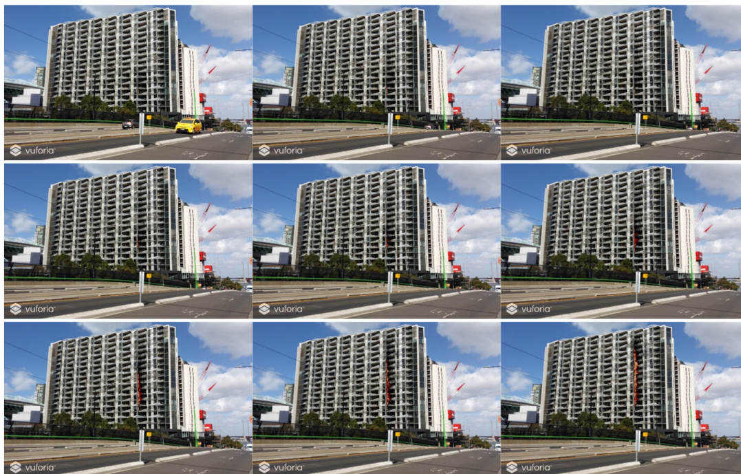
Figure 7. Sequential snapshots of AR-based fire visualisation for the outdoor building cladding fire scenario (Case 1), illustrating the simulated fire spread progression from 6 to 238 s. The AR overlay, using Vuforia-based tracking, aligns the virtual fire dynamics with the real-world structure to enhance situational awareness.
