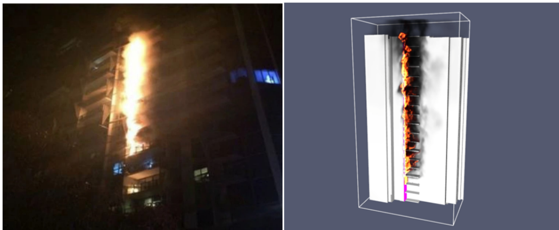
Figure 6. A comparison between a real-world image of the Lacrosse Building fire in Melbourne (left) [39] and an FDS simulation at 250 s (right). Both illustrate the rapid vertical flame spread along the building façade, primarily driven by the combustible aluminium composite panel (ACP) cladding. The simulation effectively captures the fire dynamics observed in the actual incident, highlighting the role of façade materials in fire propagation.
