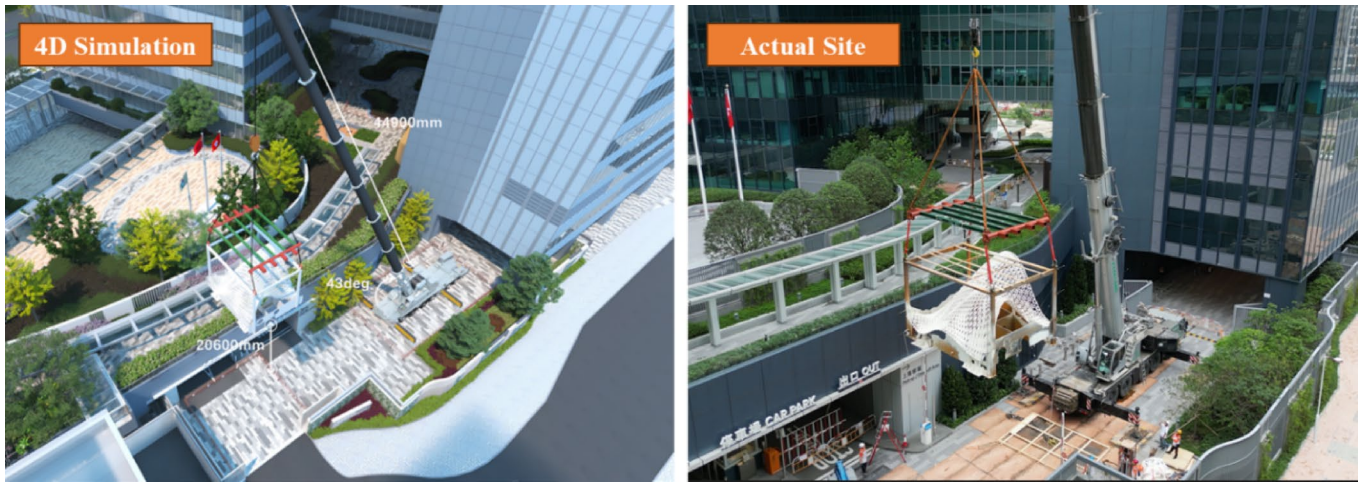
Fig. 25. 4D simulation (Virtual) and Actual Single-day installation (Reality).
