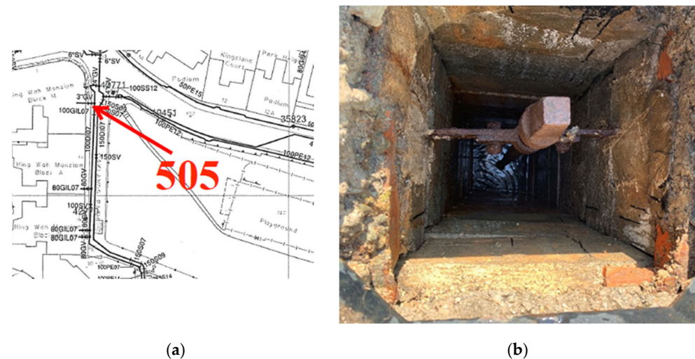
Figure 3. (a) Typical installation points for noise loggers in real water distribution pipeline, and (b) typical leak location.
