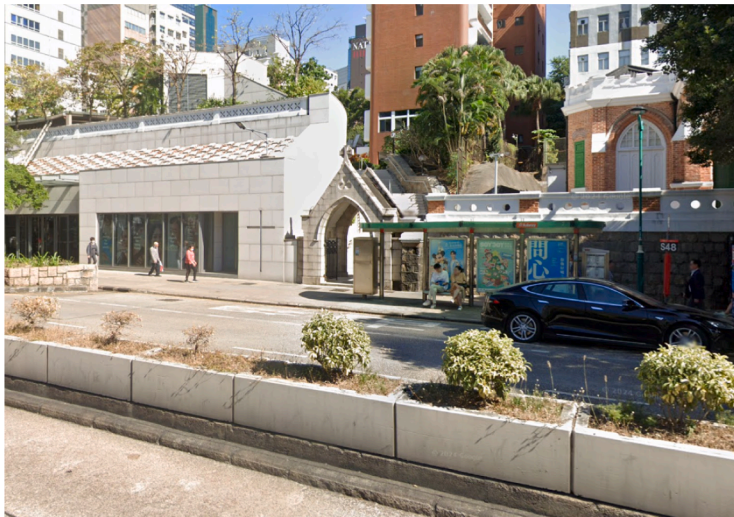
(a) An example of green strip in an existing road in Hong Kong
