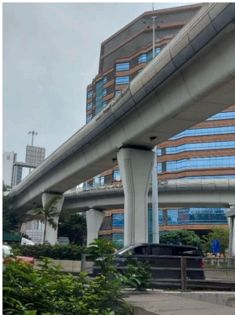
(c) Elevated highways in Hong Kong
