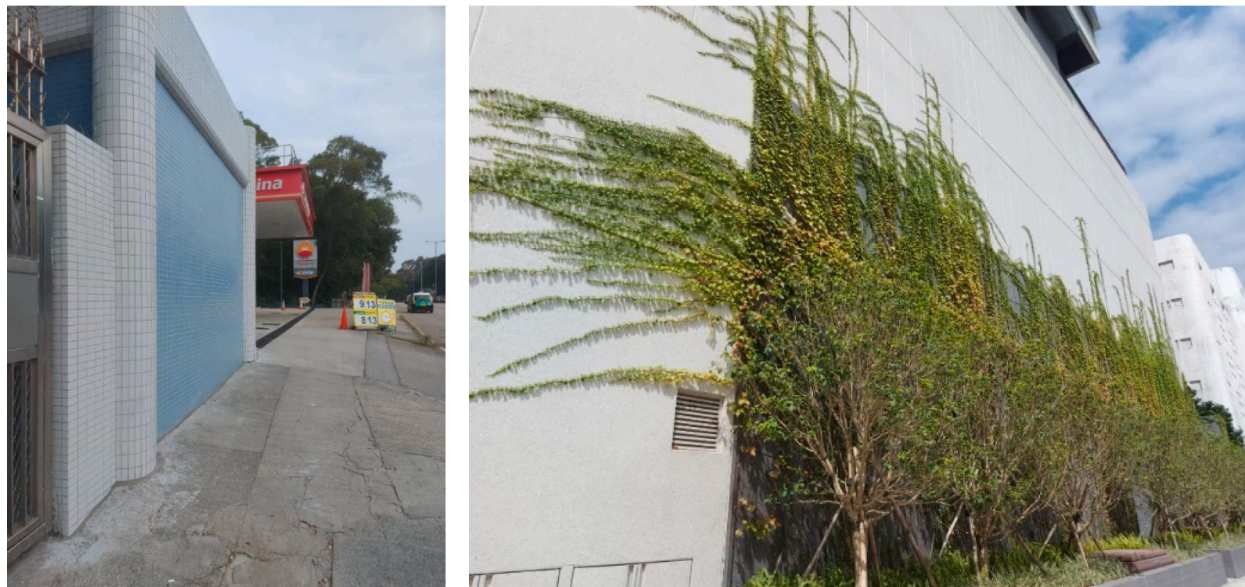
(a) A typical wall of a building on the street
