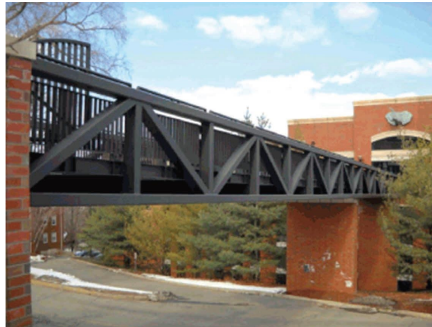
FIGURE 11: Dowling Hall footbridge [34].
