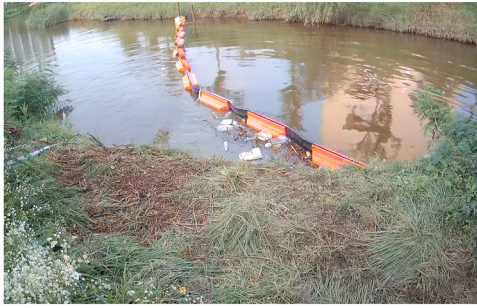
Fig. 1. A floating barrier on the river to collect plastic waste and debris, preventing pollution from spreading downstream.
