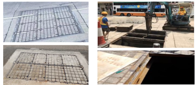
(a) MPCs on the road (b) Manually inspection with road closure Fig. 1 MPCs and the costly manually inspection
