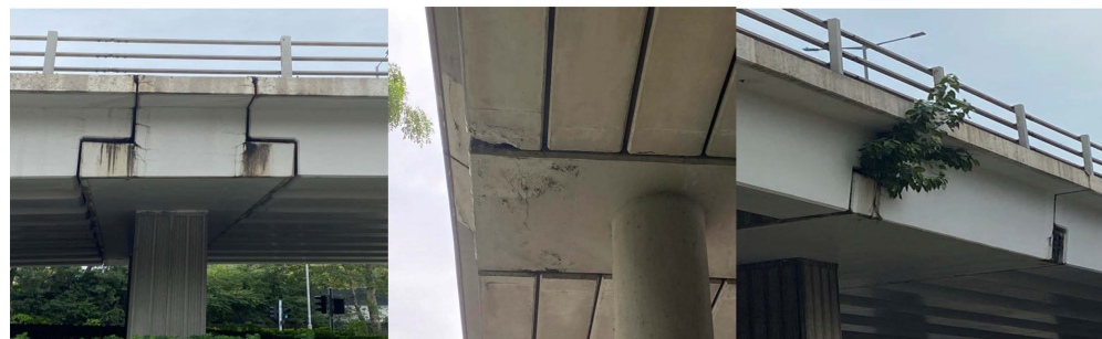
Figure 16. Deterioration at the bridge joints caused by rain and vegetation.
