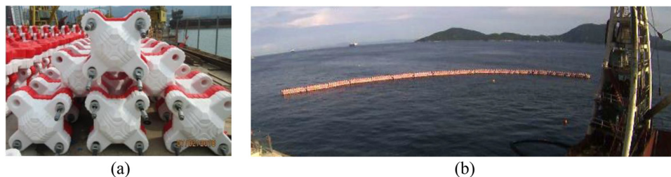
FIG. 1. (a) Physical model of the FB, WhisprWave, (b) an illustrative case implemented near a seawall in Hong Kong (Courtesy of the Drainage Services Department, Hong Kong Special Administrative Government).
