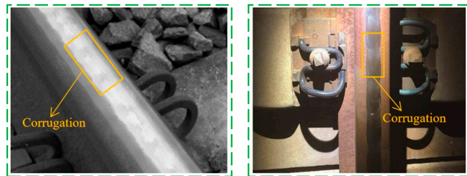
Figure 1. Schematic diagram of rail corrugation.
