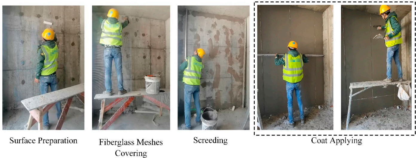
Figure 7. Typical operations of each task in plastering work.
