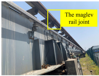
Fig. 7. Maglev rail joint on the straight segment of Shanghai Lin-Gang maglev test line.
