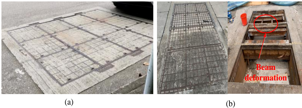
Fig.9 MPC: (a) normal; (b) fault
