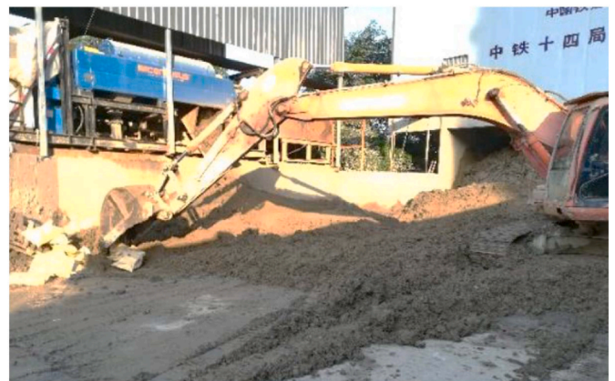
Fig. 15. Stockpiling of discharged soil from shield tunnel construction (Zhang et al., 2022a).
