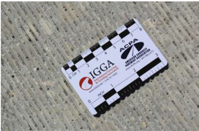
Fig. 5. Concrete surface immediately after grinding.
