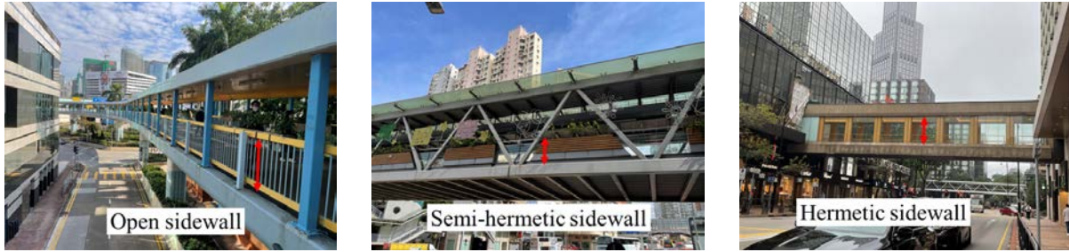
Fig. 1. Some elevated walkways in Hong Kong photographed by authors.
