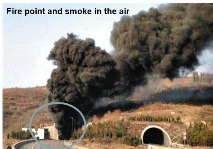
Fig. 12 Jinji Road Tunnel fire in 2014[101].
