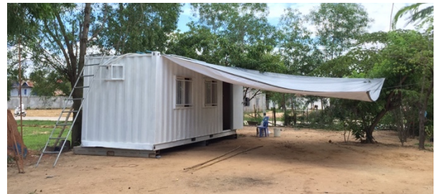
Fig. 2 Delivery of the second-hand 20-foot shipping container
