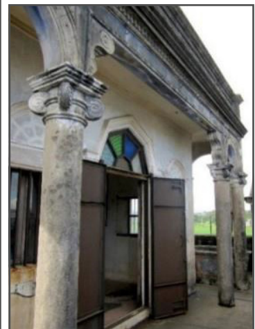
Fig. 2.29 The retreated (modified) Ionic colonnade on the 7th floor of the Rui Shi tower, Kaiping 37
