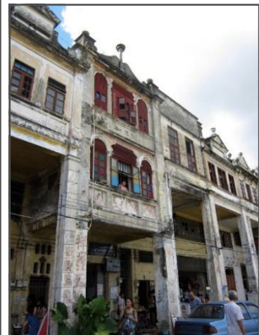
Fig 2.23 Aligned arcade buildings on West Embankment Street, Chikan Ancient Village, Kaiping 31
