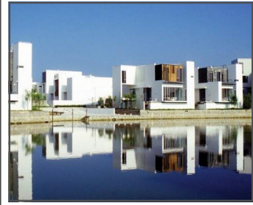
Fig.2.37 The Boao Canal Village houses, Hainan, China 46
