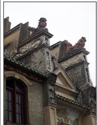
Fig 2.32 Gable walls of Feng Chai Ancestor Hall, Kaiping 40
