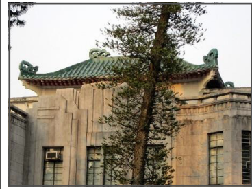
Fig. 2.13 Stylistic adaptive approach: Morrison Building of Hoh Fuk Tong, Tuen Mun, Hong Kong
