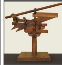
Fig 2.4 & 2.5 Chinese Dougong Column detail. 9 10
