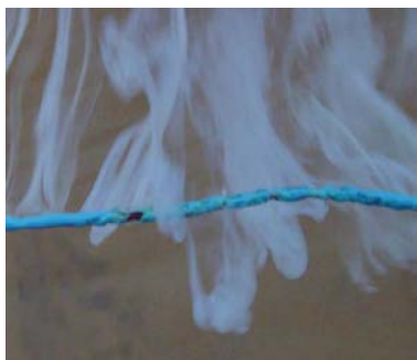
Figure 2. Combusting of insulation material due to overload
