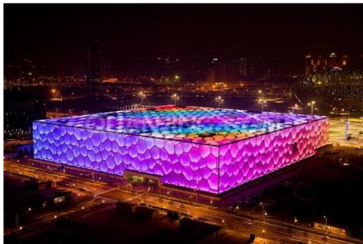
A: The Water Cube, Beijing, China
