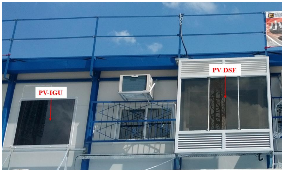
Fig. 2. PV-DSF and PV-IGU on the south-facing façade of the site office building.
