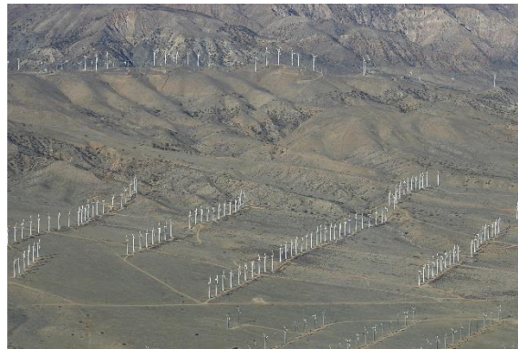
Figure 3 Aerial view of the Tehachapi Pass Wind Farm [17]
