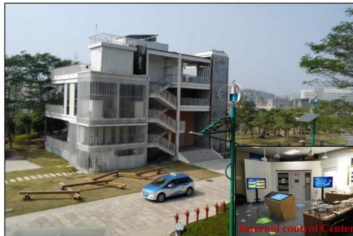
Fig. 2 Low-energy building installed with the PV-BES system in Shenzhen
