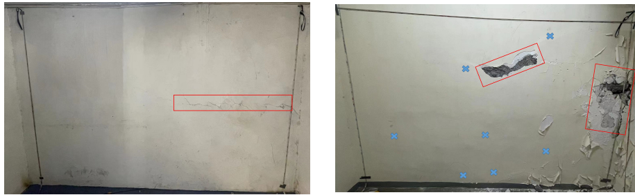
Figure 3: The upper deck (left) and the lower deck (right) of the Tuen Mun wall. The red boxes indicate the surface defects and the blue crosses indicate locations with debond.
