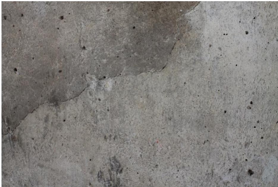
Figure 5. Image of cracks on the Hsichou Bridge
