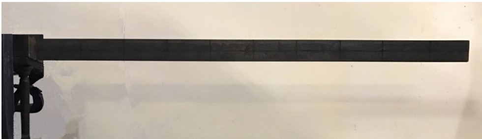
Fig. 2. Overview of the beam structure
