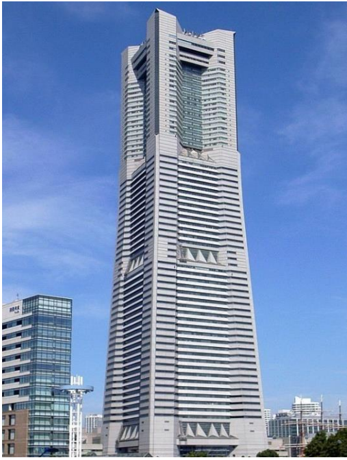
(a) Landmark Tower, Yokohama (600 MPa) [4]
