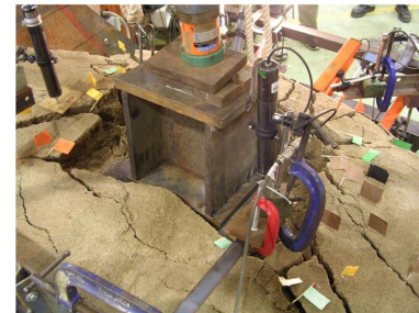
(e) Penetration of base plate into the soil
