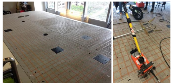
Figure 1 Glass-fibre panel pavement in Underground Utility Survey Lab, PolyU and 900MHz GPR system
