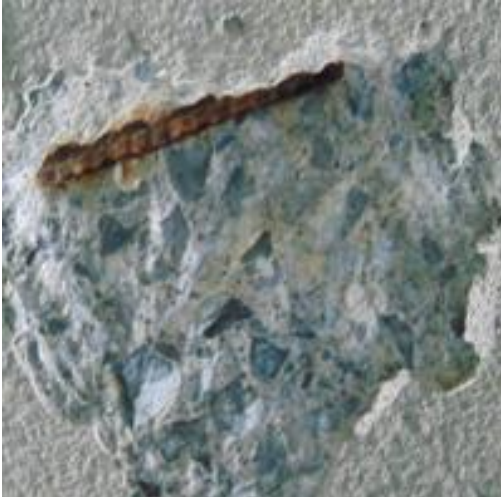
(a) Spalling -Image “A”
