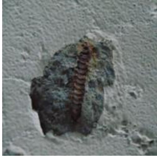
(b) Spalling -Image “B”
