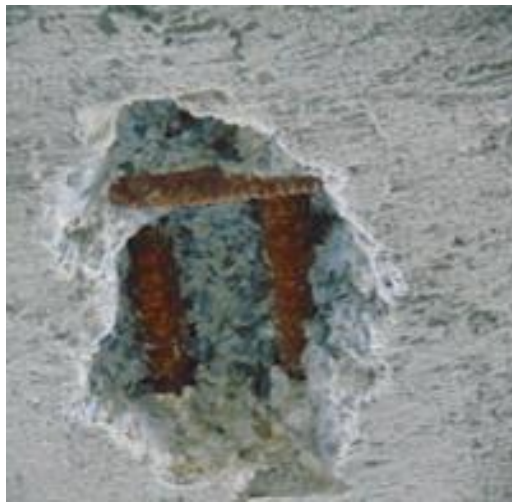
(c) Spalling-Image "C"
