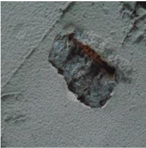
(c) Spalling-Image “C”
