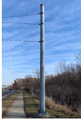
Fig. 1. Use of octagonal hollow section (West Lafayette, US).
