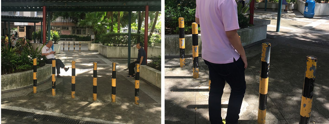
Figure 4. Bollards were installed in front of the main entrance, which not only segregated wheelchair users but also created a dangerous condition for the visually impaired
