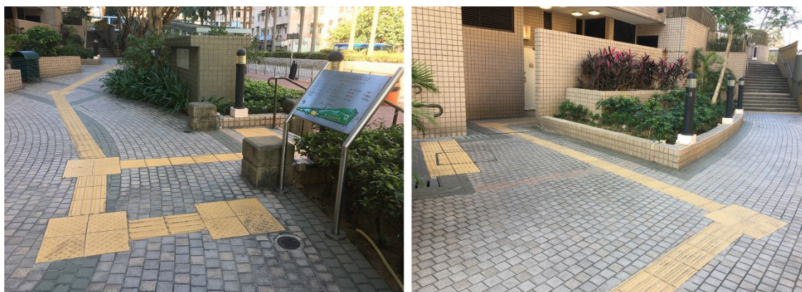
Figure 5. Comprehensive tactile paths were paved to provide guidance to visually impaired persons
