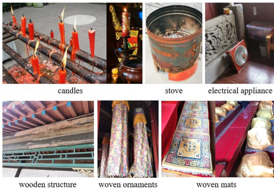
Fig. 1. Typical fire hazards in Chinese historical buildings.
